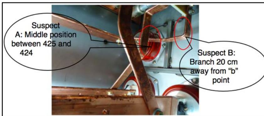
Figure 12. Suspected PD source location
